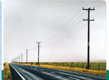
Power Distribution Line Insulators
